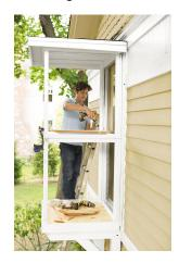
the lower one with 2½-inch screws every 10 inches, but don't seat them fully just yet. Use 1 5⁄8-inch screws to attach 1x4s to the back edges of the joined frame, between the trim boards, to pad out the window casing. Drive 3-inch deck screws through the lower frame's plywood supports and into the brackets. Add the floor and screw it to the supports.
